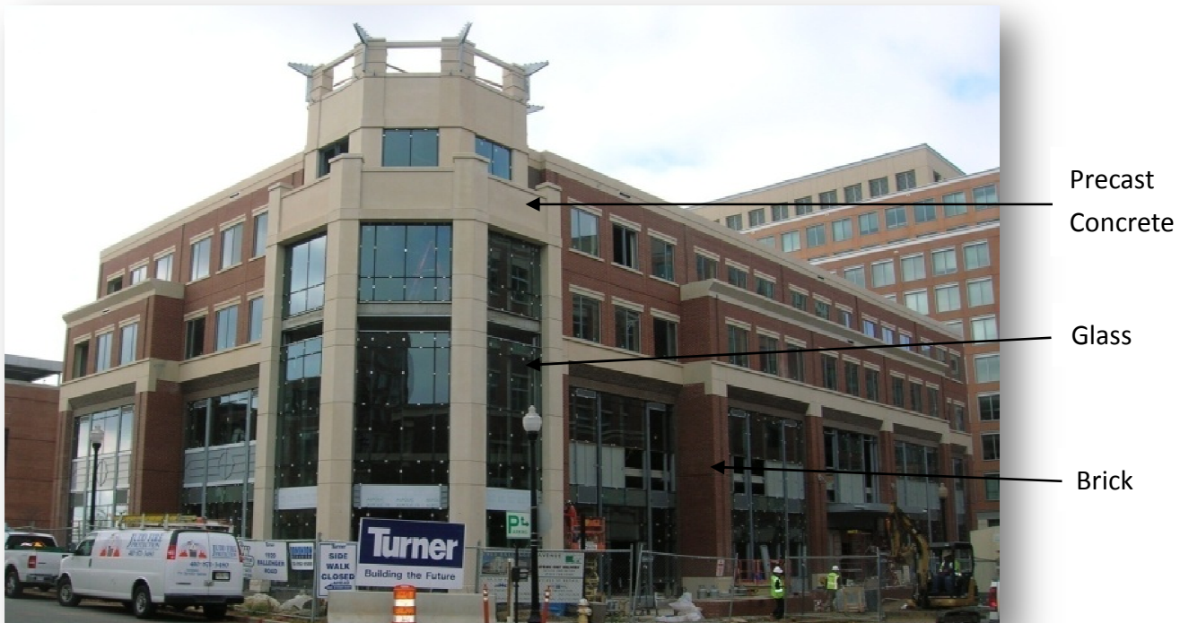
[Figure 1 – major materials on the facade]
